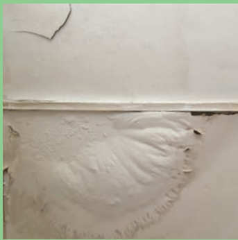
Water leakages
