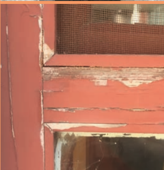
Exterior wood protection issues (peeling paint, lack of varnish /oil)
