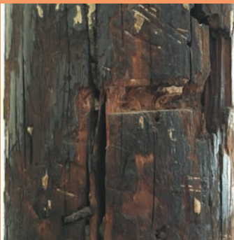
Wood cracking
