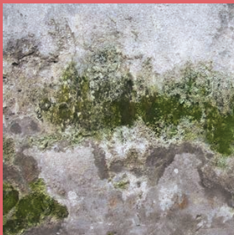
Exterior walls humidity
