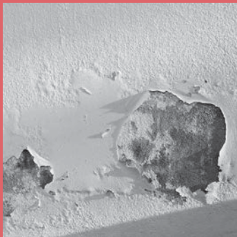
Falling plaster, peeling paint, air bubbles
