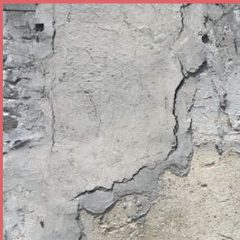
Falling plaster, peeling paint, air bubbles
