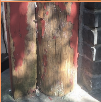
Exterior wood protection issues (peeling paint, lack of varnish /oil)
